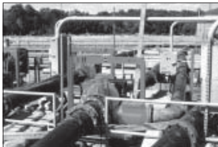
Wastewater Treatment Plant Bypass Project – Temporary installation of twelve 12" (300mm) DPC300 electric drive Dri-Prime pumps
