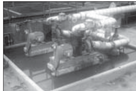
API Separator Sludge Removal – Permanent installation of two 6" (150mm) CD150M electric drive Dri-Prime pumps
